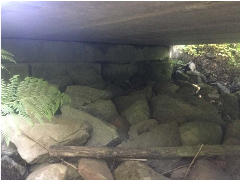
Left Bank Abutment when facing downstream
