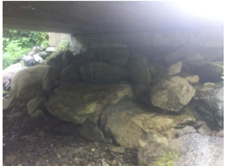
Right Bank Abutment when facing downstream
