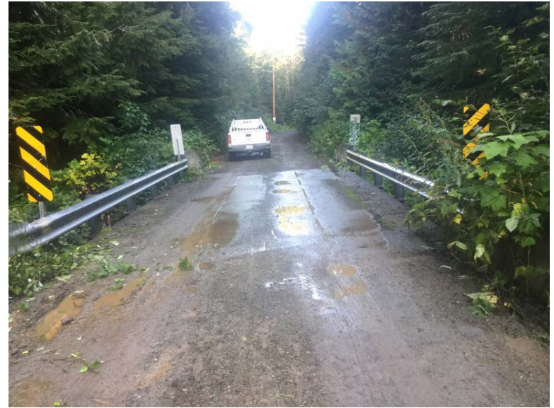
Approach from Right Bank when facing downstream
